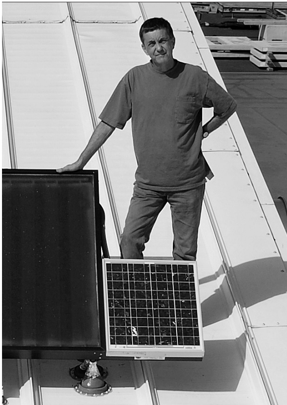
Warehouseman Earl Ayers oversaw the remodel of the PUD offices and facilities, including the installation of this solar heating system that provides hot water to the buildings.
